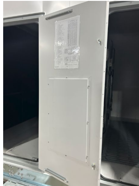
FIGURE 2: LOCATION OF BLOCK-OFF PANELS BEHIND THE DOOR.
