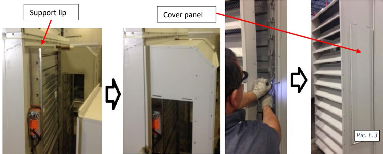
**Outdoor AND Indoor Dehumidifier - Field-installed OA (outdoor air intake) Filter Rack Installation**
